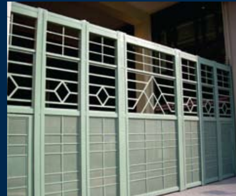
Lazarus Department Store Columbus, Ohio Custom Vertical Lift Doors
